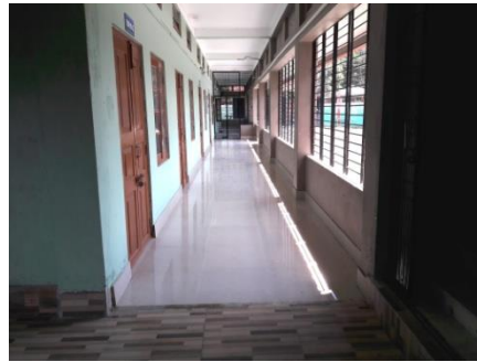
Ground floor protected by grills
